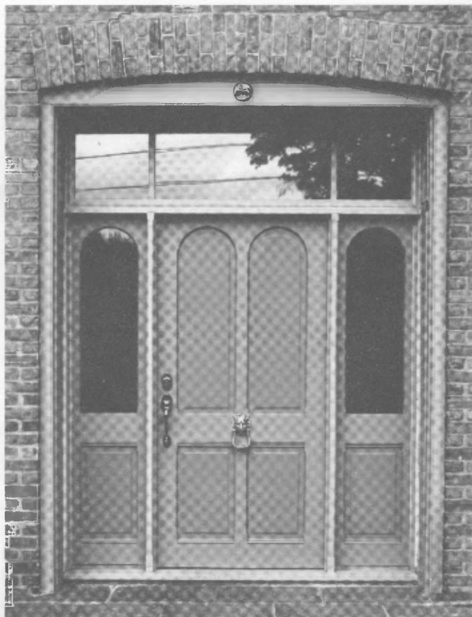
Michael Cleary of Arran Township has crafted a fine replacement main door for the old Lodge building.
